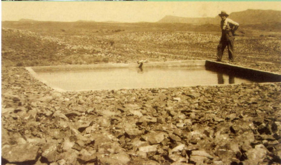
BELOW: Joseph Archer standing alongside the reservoir at Whitehill in 1927. Photo: SANBI Collection.
