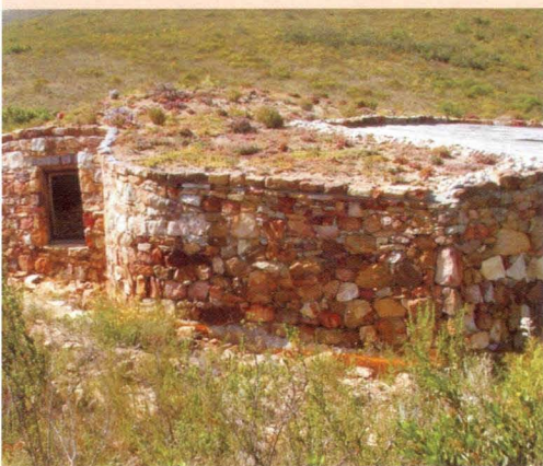
TOP: The Towerland succulent roof garden with the Langeberg in the background. ABOVE: Melting into the background. Towerland Wilderness Retreat fits harmoniously into the landscape, creating a fireproof roof which is a major consideration in the fynbos-covered mountain area. Photos: Ernst van Jaarsveld.
